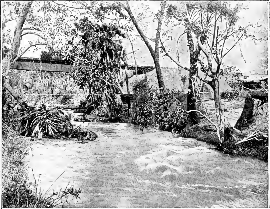
"THE RIVER CROSSED BY MEANS OF A TEMPORARY BRIDGE."
